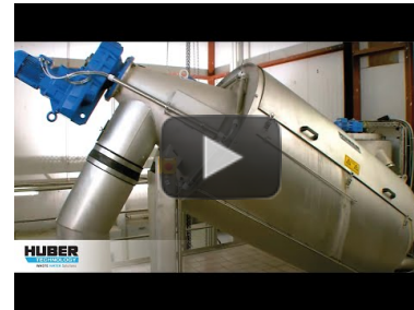
Video: HUBER Screw Thickener S-DRUM (RoS2) - here at a municipal WWTP https://www.youtube.com/watch?v=uxjMve6yi50
