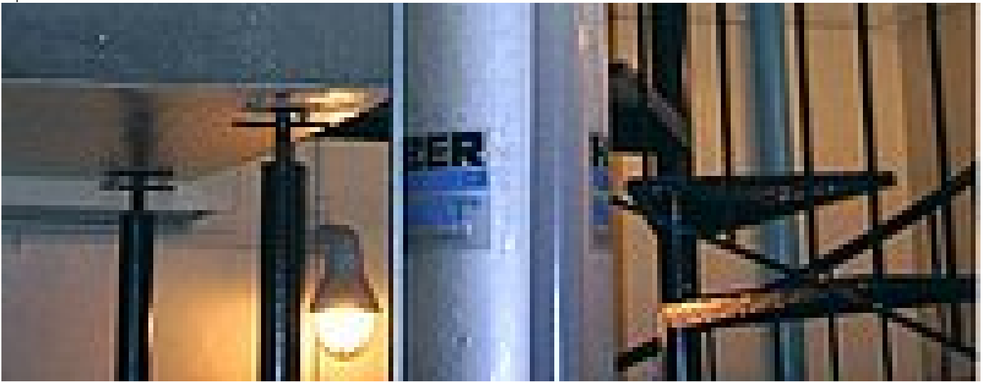
Vertical screenings transport tube of the RoK 4
