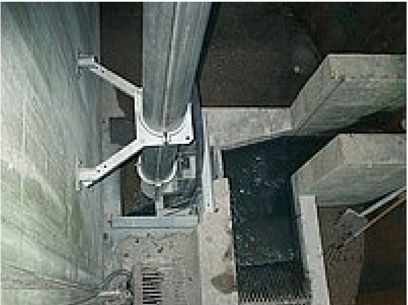
Lower section of the RoK 4 with screen basket and IRGA for screenings washing
