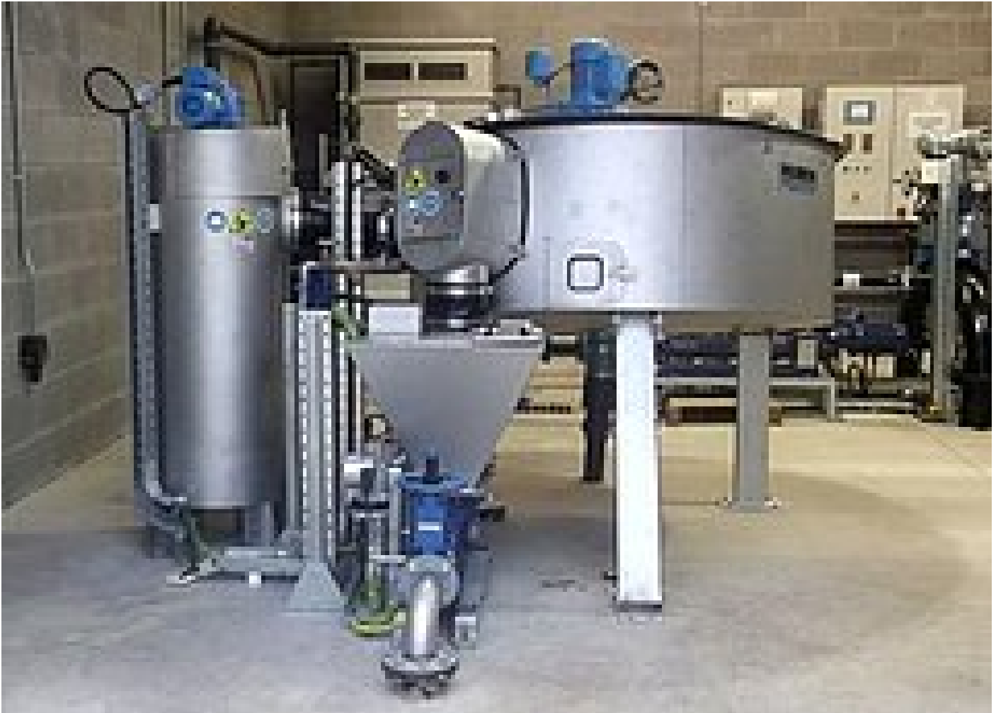
HUBER Disc Thickener S-DISC at Magilligan WwTW
