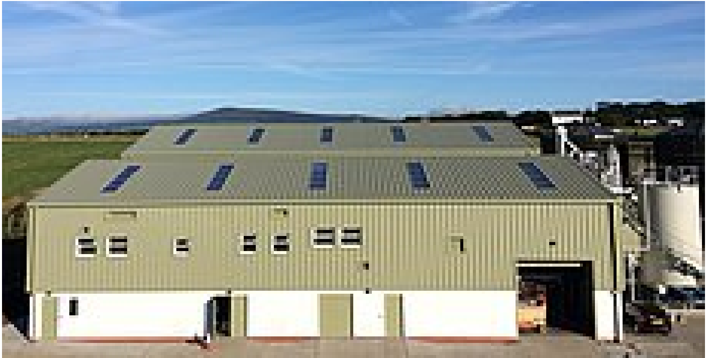
Exterior view of the drying hall
