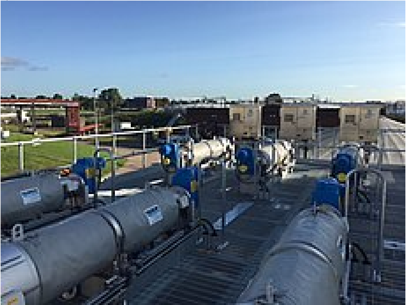
Minworth STW STRAINPRESS® Installation
