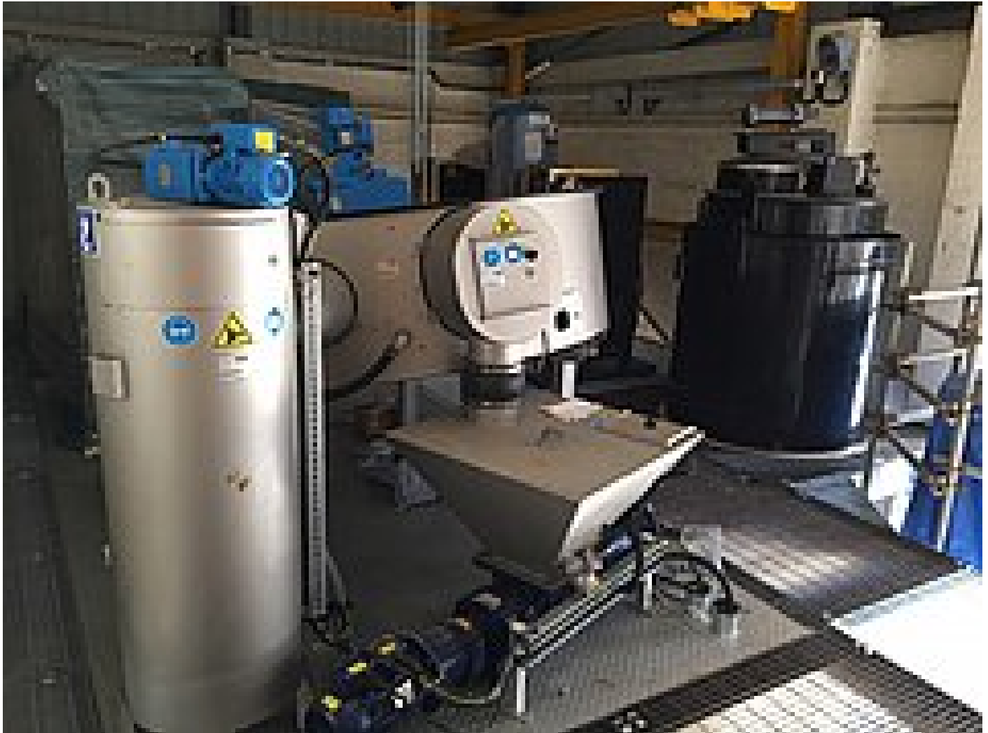
Installed HUBER DISC Thickener S-DISC at Great Dunmow
