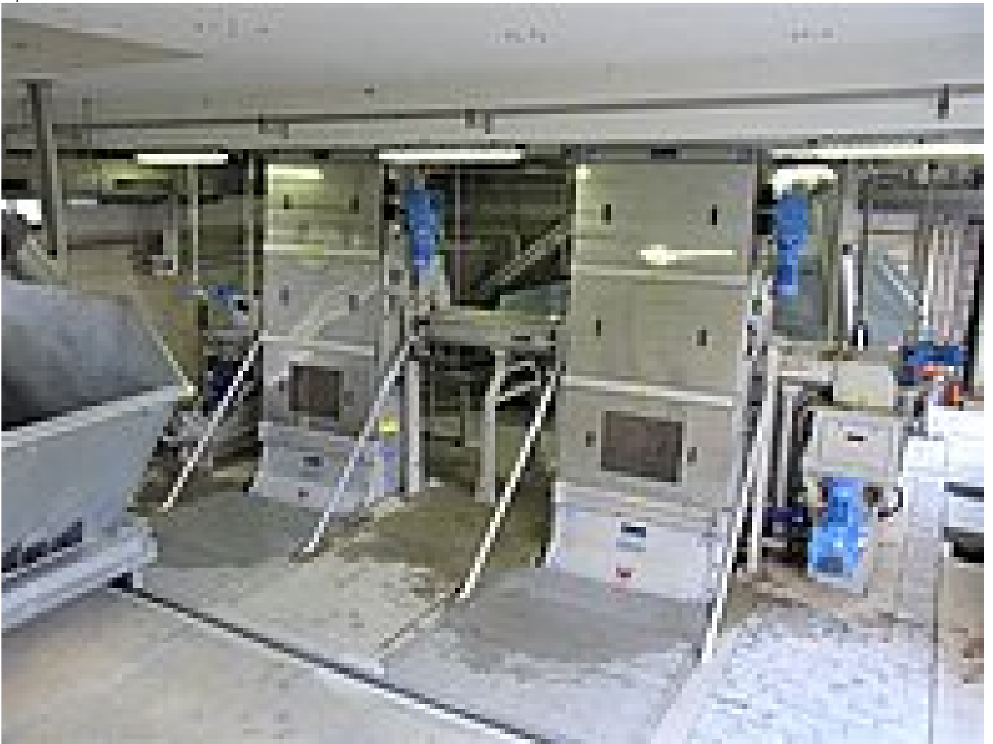
The HUBER Multi-Rake Bar Screen RakeMax® HF with its cranked frame construction is almost indistinguishable from the proven basic RakeMax® machine from the outside.
