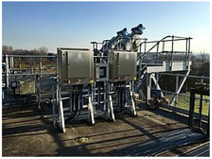
Huber Technology completed the inlet screen upgrade at Pulborough STW, installing two HUBER Micro Strainer ROTAMAT® Ro9 / 700's on an elevated inlet works.
