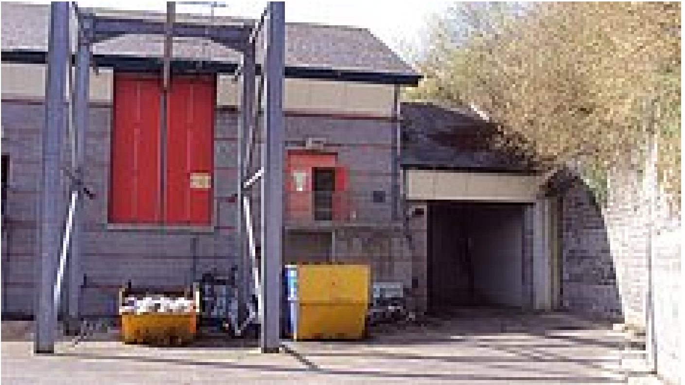
Outside access to site and large door access to Inlet Works
