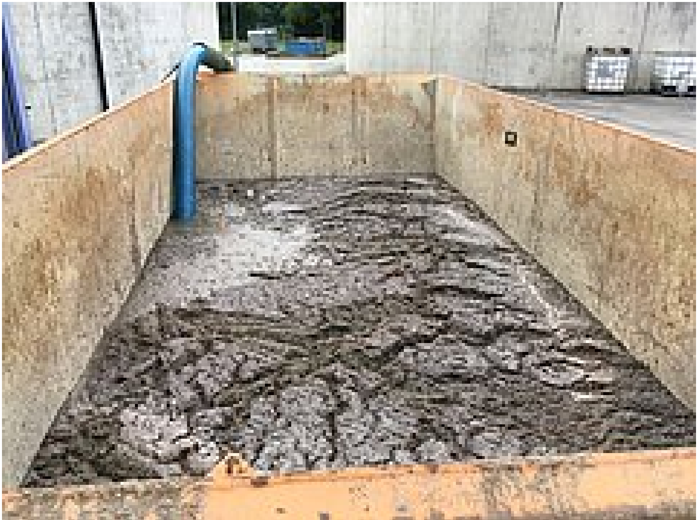
Fig. 3: Thickened primary sludge from the HUBER Drum Screen LIQUID demo unit after a HUBER Disc Thickener S-DISC
