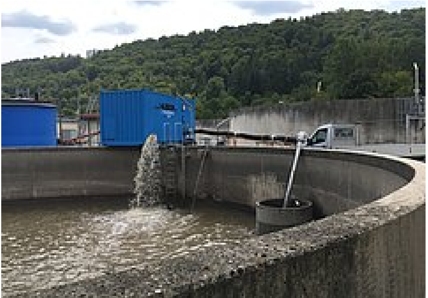
Fig. 1: Validation operation - a pump sump was retrofitted into an existing buffer tank with concrete shaft segments. The demonstration plant HUBER Drum Screen LIQUID is fed with the effluent from the mechanical pre-treatment system. The effluent (screened wastewater) of the LIQUID machine flows by gravity back into the buffer tank
