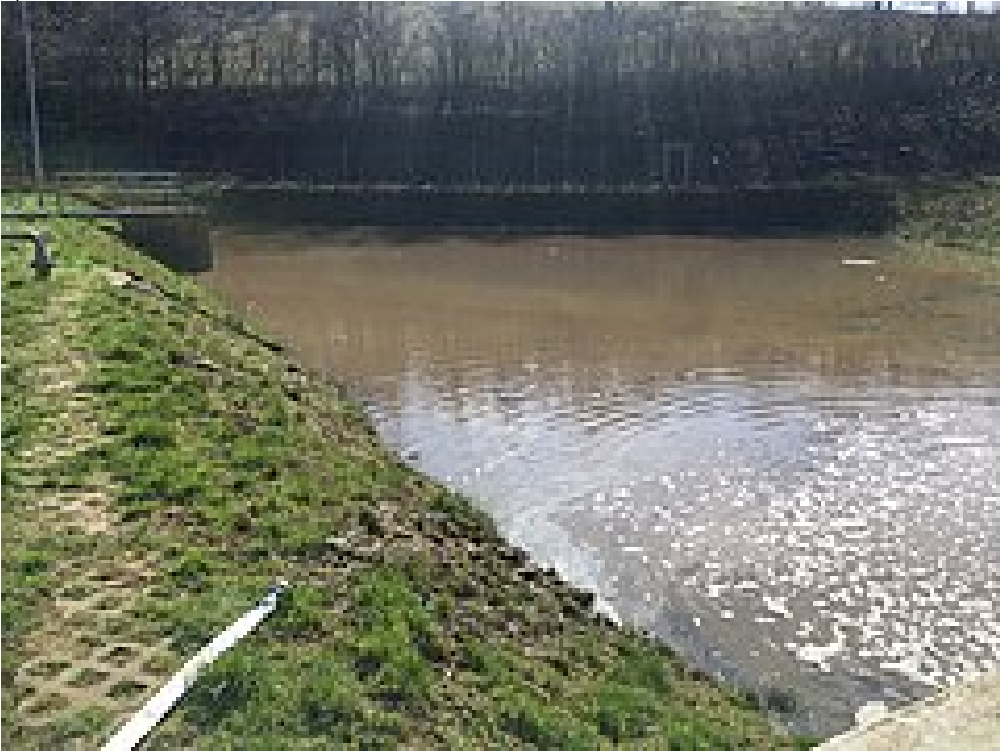
Fig. 6: Bridging operation - polishing pond converted into a settling pond for static thickening of the thin sludge from the HUBER Drum Screen LIQUID demonstration plant
