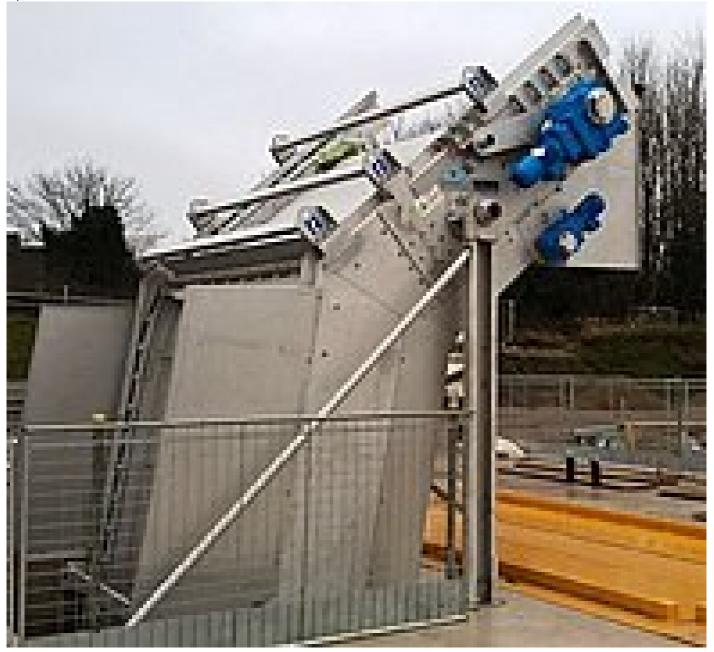
HUBER Technology recently supplied three HUBER Coarse Screen TrashMax® heavy debris removal screens to a site in the North West of England, which is one of the largest wastewater treatment plants in the UK. These are the first screens of this design to be installed anywhere in the UK.
