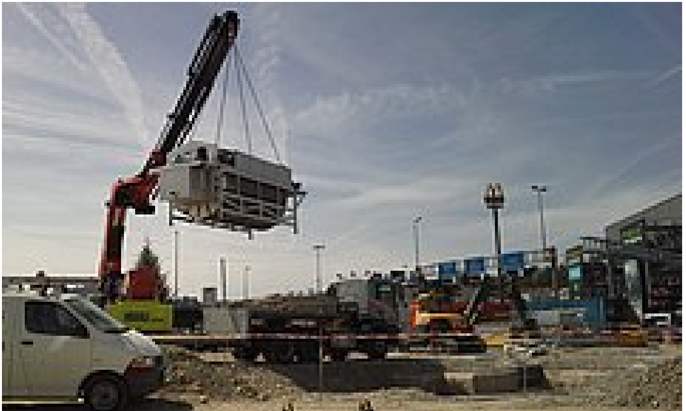
Installation of the road runoff treatment plant under a roundabout
