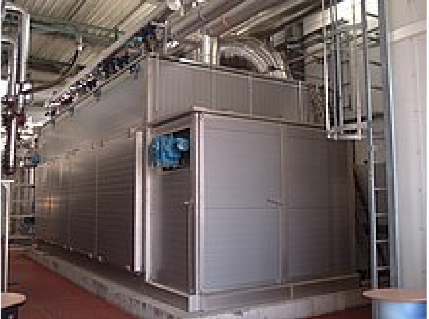
Middle temperature sewage sludge drying with HUBER Belt Dryer BT
