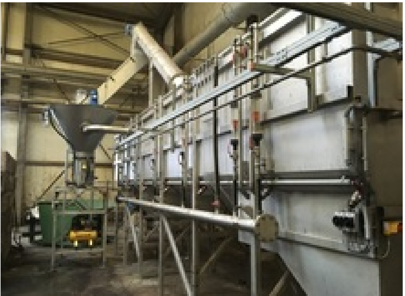
Fig. 1: HUBER Longitudinal Grit Trap ROTAMAT® Ro6 Bio (right) with downstream HUBER Grit Washer RoSF G4E (left)
