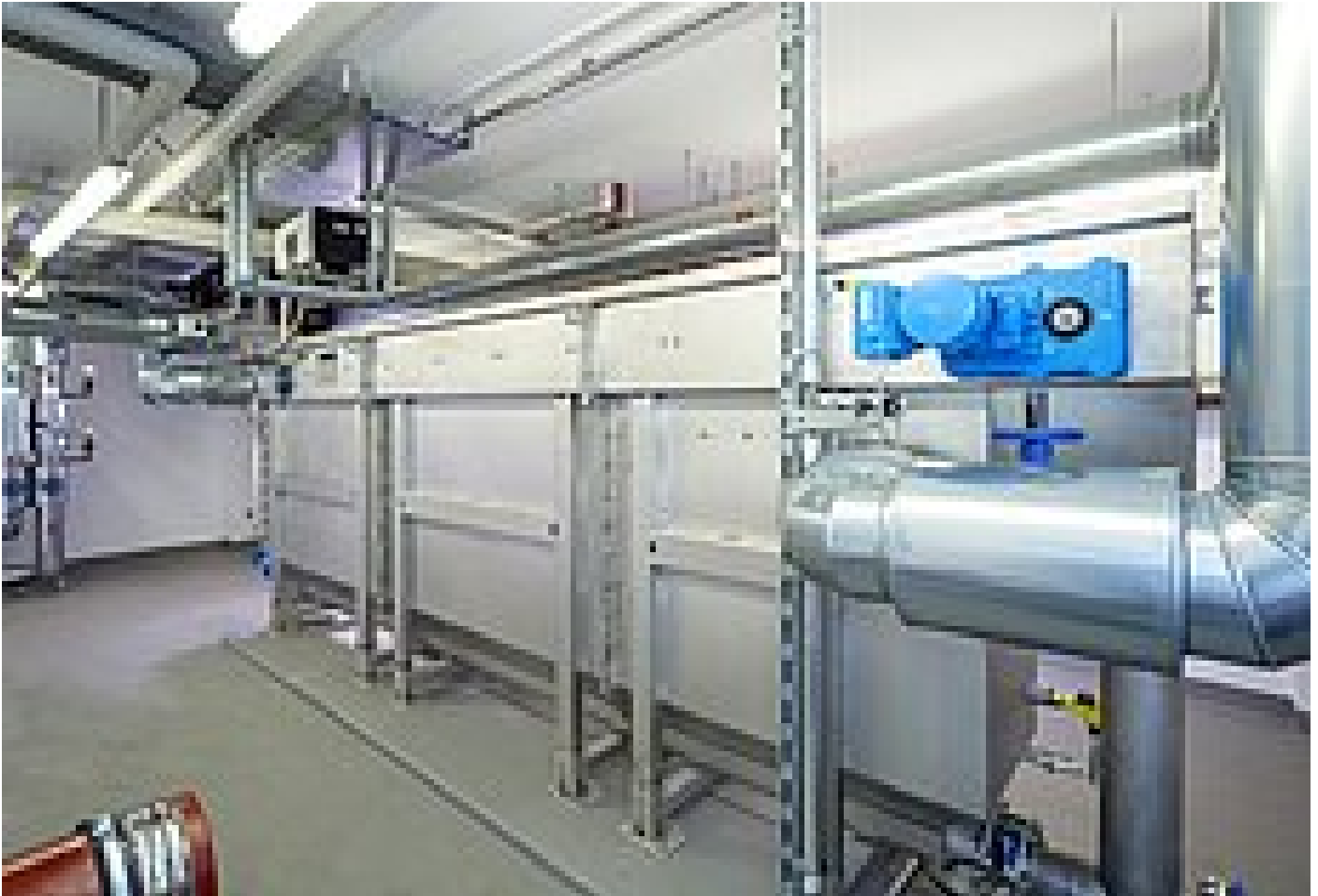
Flanged version of a HUBER RoWin Heat Exchanger, optimally installed in a confined space.
