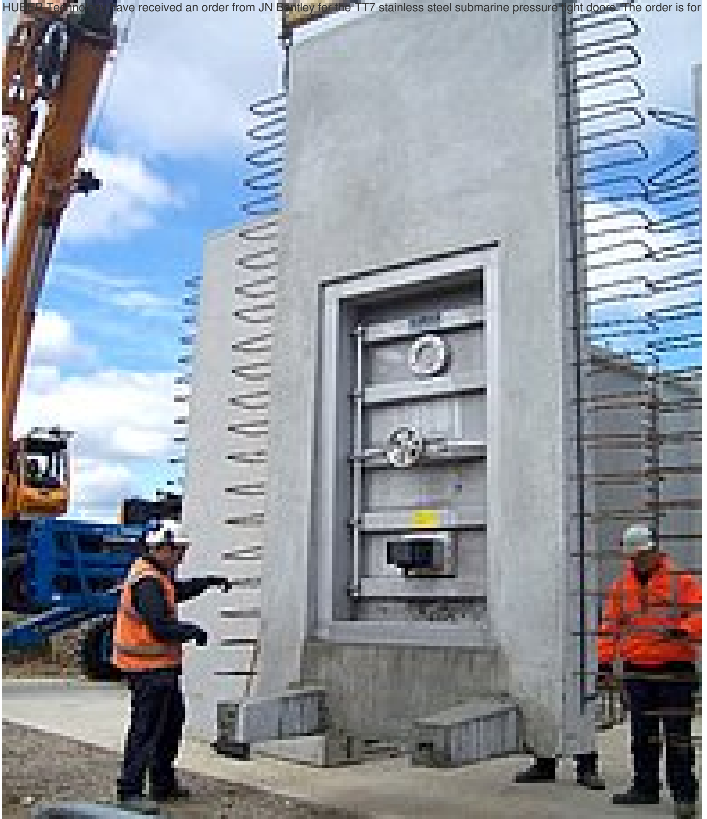
HUBER TT7 pressure tight stainless steel submarine door
