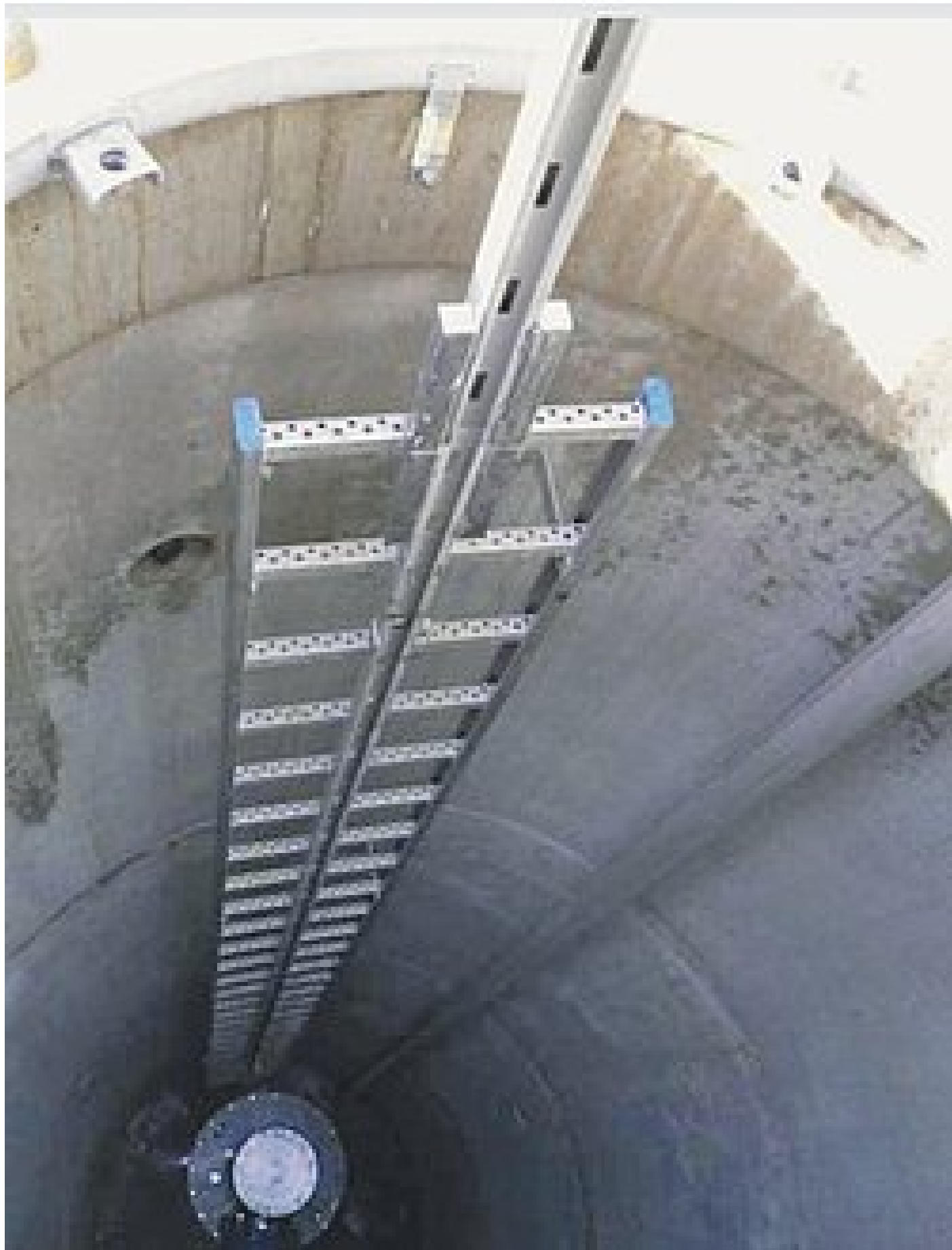
Safe access: ladder with safety guard rail
