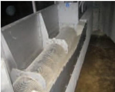
ROTAMAT® Storm Screen RoK 2 combined with discharged flow volume measurement
