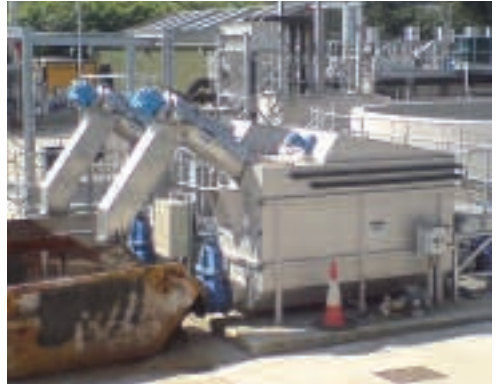
ROTAMAT® Membrane Screen ideal for removal of hairs and fibres
