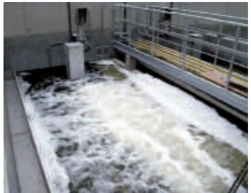
VRM® unit installed on municipal WWTP Hutthurm, 3 VRM® 30/544 units, 9.792 m 2 membrane surface
