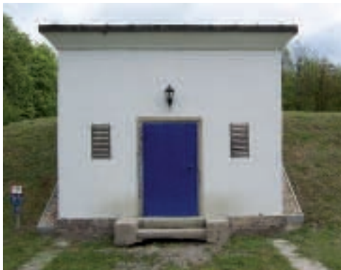
Drinking water reservoir with HUBER equipment
