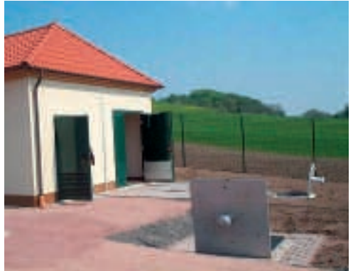
MCB unit (size 150 PE) for decentralized wastewater treatment in a biosphere reserve
