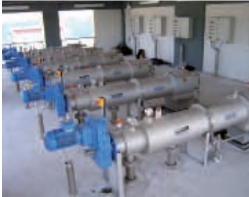
STRAINPRESS® – continuous pressurised coarse material separation
