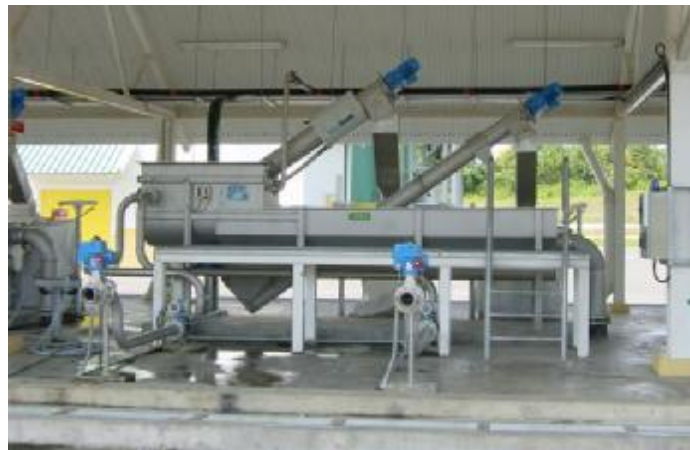
HUBER Sludge Acceptance Plant Compact Ro 3.3
