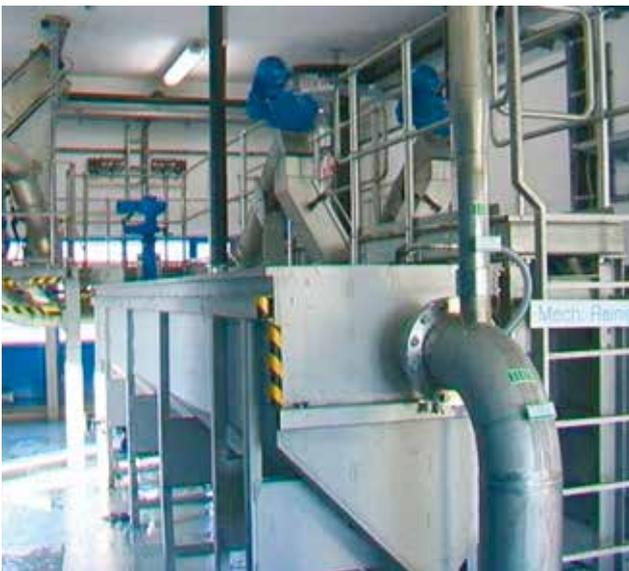
Above-ground redundant installation of a HUBER Longitudinal Grit Trap ROTAMAT® Ro6.
