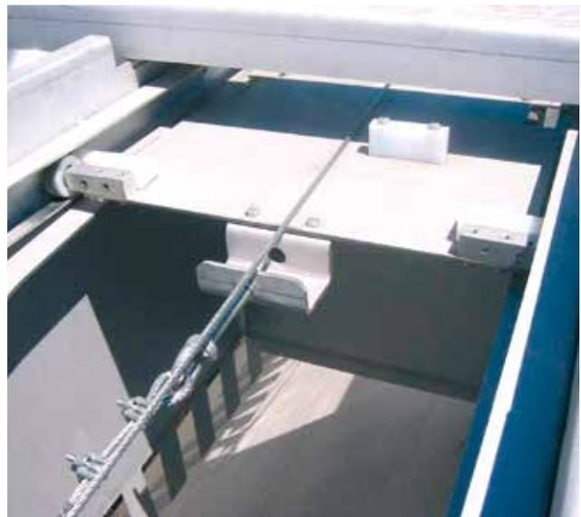
Automatic grease removal by means of a paddle system.
