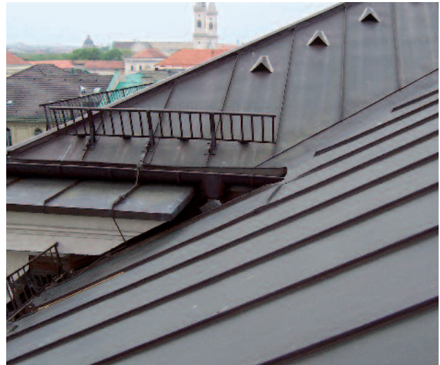
Copper roof with a patina
