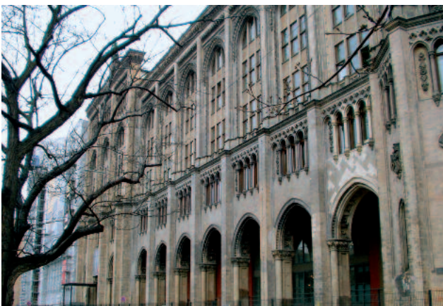
Government building in Munich Roofage A_{red} = 1800 \text{ m}^2
