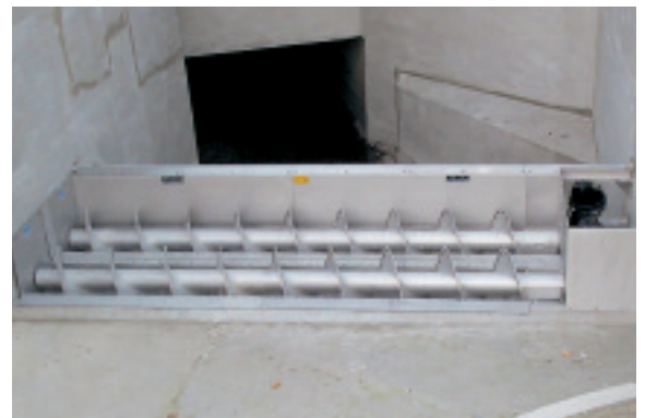
Twin screen for high flows over short weirs
