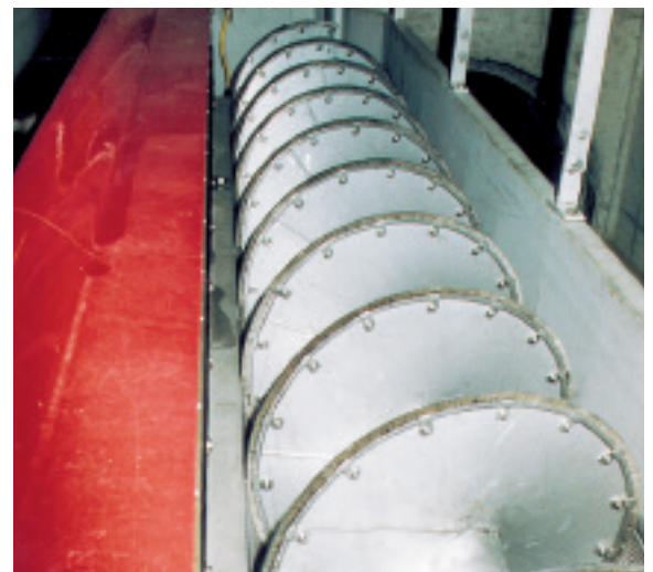
Screw with cleaning brush in horizontal 28" (700 mm) diameter trough attached to the downstream side of an overflow weir
