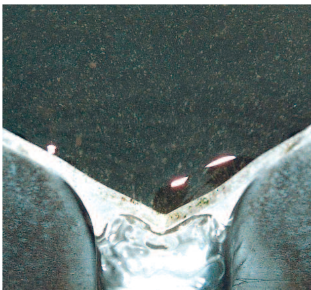
Secondary clarifier effluent with high suspended solids concentration
