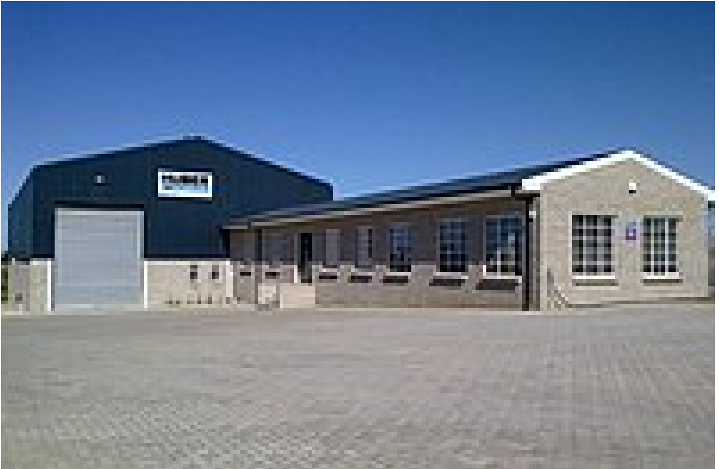
Huber Technology (Pty) Ltd head office
