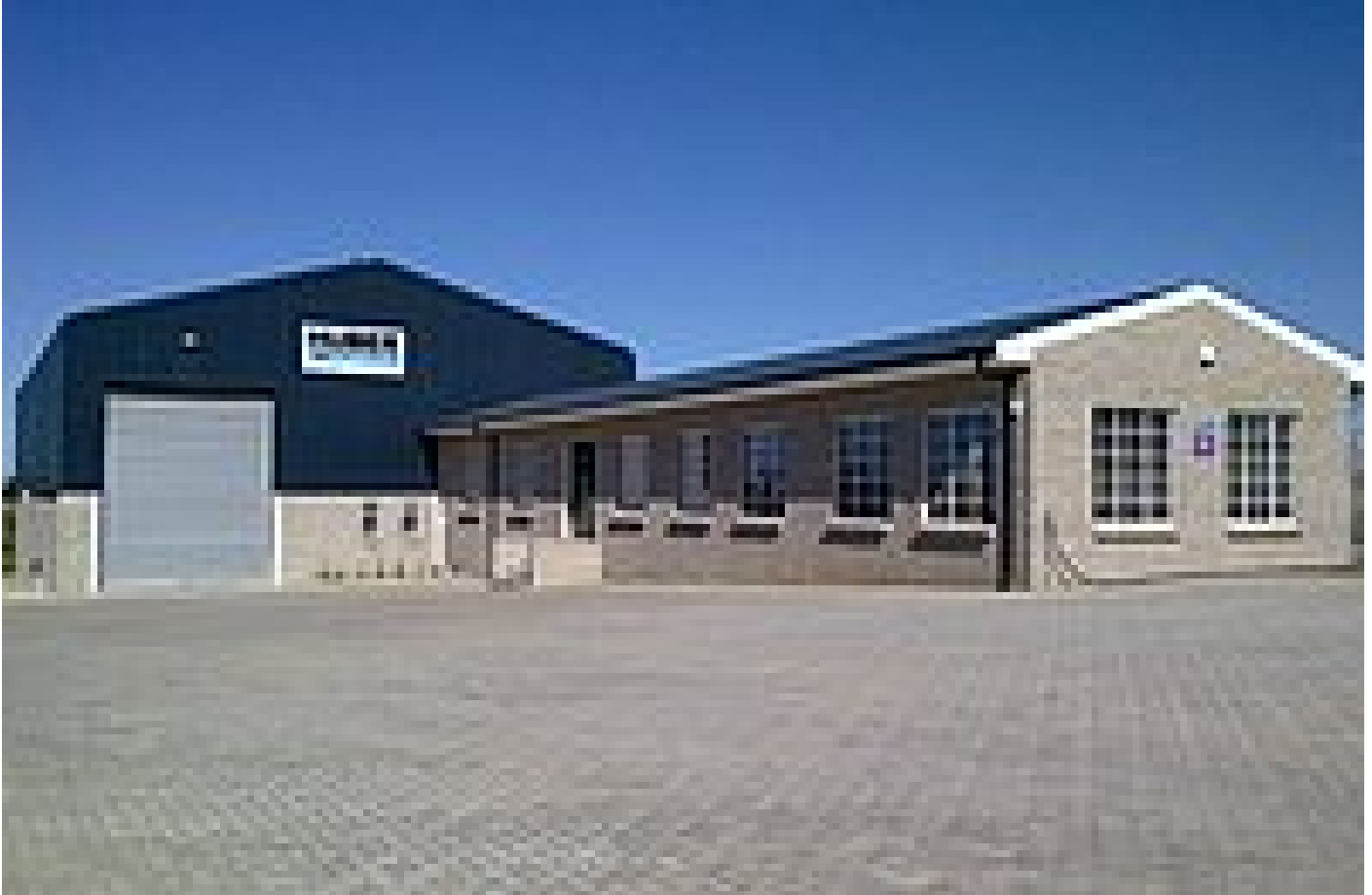
Huber Technology (Pty) Ltd head office
