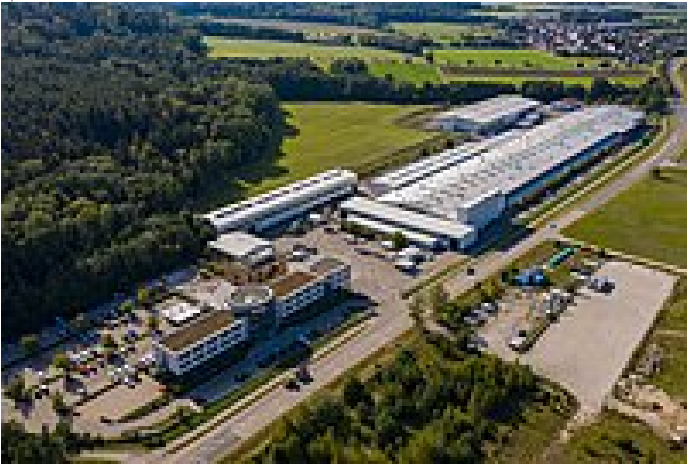
30,000 m 2 main production factory and offices of HUBER SE in Germany
